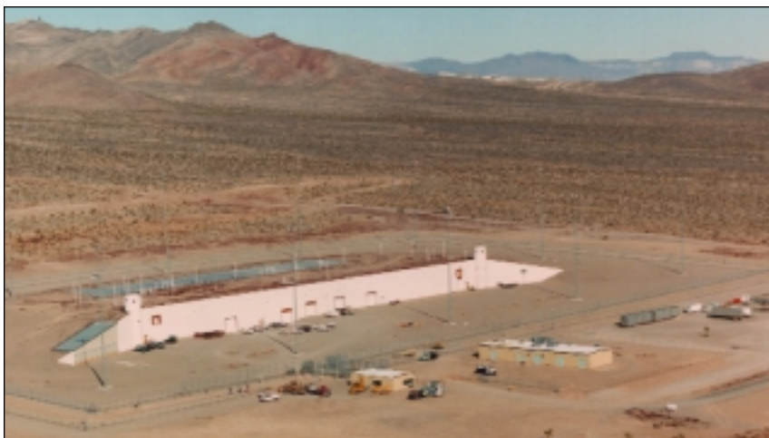
Device Assembly Facility at the Nevada Test Site.
