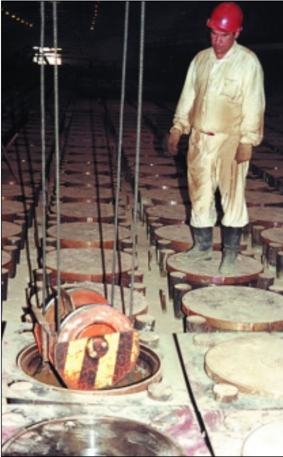
In the Mayak Storage Facility, a crane lowers the fissile material into a "nest," a cylindrical space several meters in length in which the AT-400Rs are stacked.
