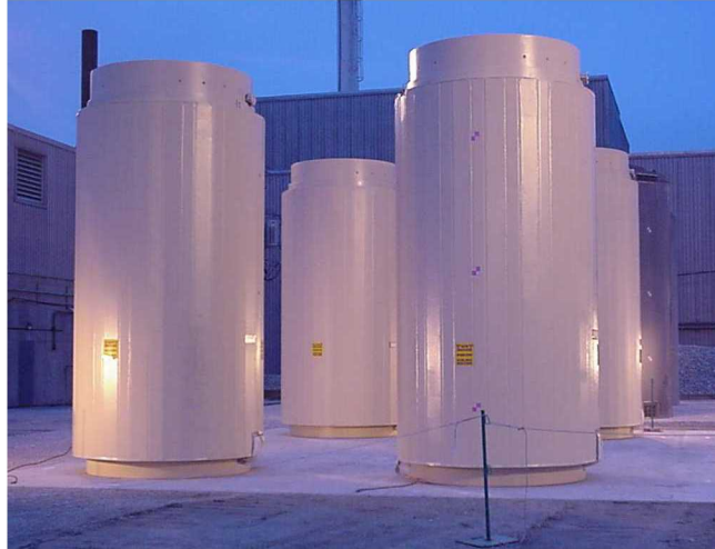
Figure 9: The HI-STAR 100 canister [20].
